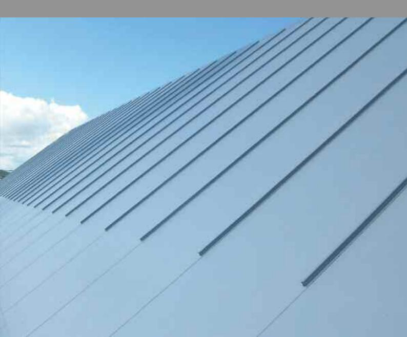
Armourplan is a PVC membrane that is produced at Clay Cross, Derbyshire, the only single-ply manufactured in the UK. It is suitable for use on a wide range of roofing applications including specialist installations such as simulated metal roofs.
